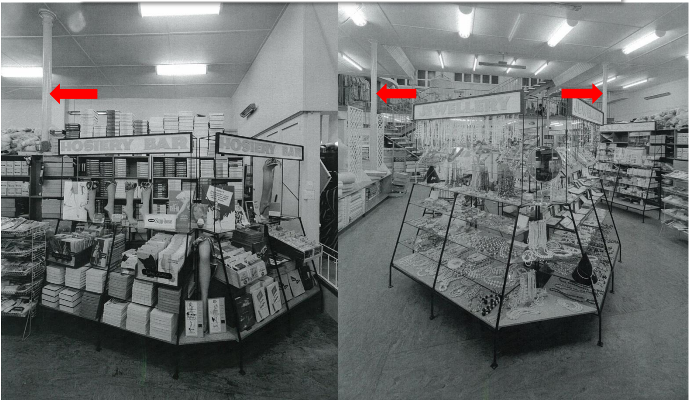
Cast iron pillars that support the 1 st floor
