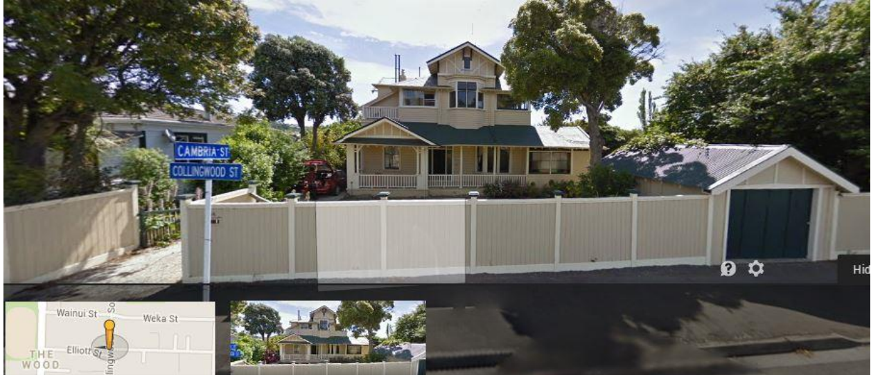
Ben and Ellen Trathen's family home, Waratah, at 10 Collingwood Street, extension by A R Griffin
