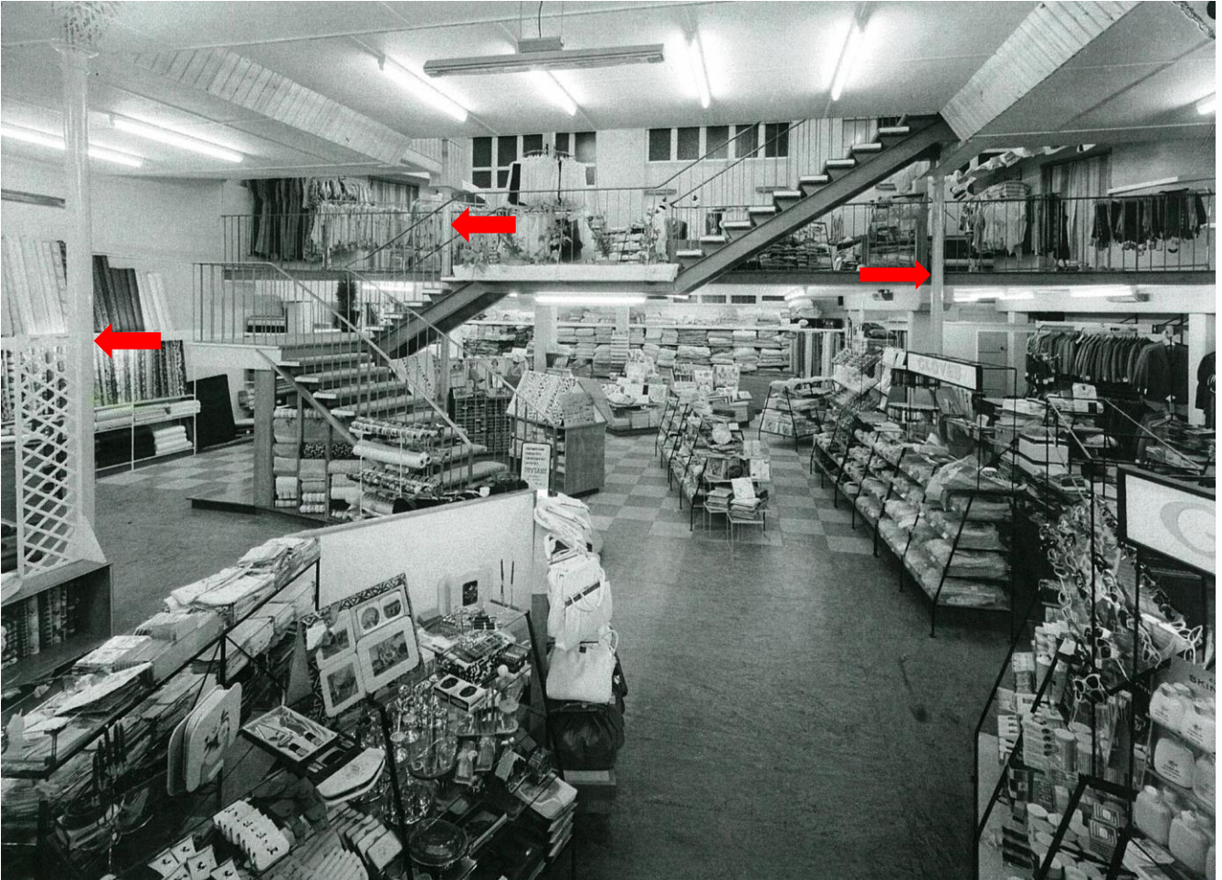
The central staircase leads to the mezzanine floor, and then continues to the second floor. Red arrows showing 1 st floor cast iron support columns
