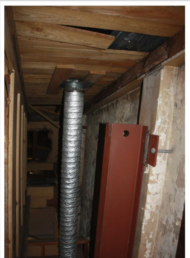
Above left: RSJ beam holding together a crack in the party wall that is shared by the Pascoe's building Above right: RSJ beam on party wall. Note it does not go to the top of the wall and the parapet extends another metre above the roof.
