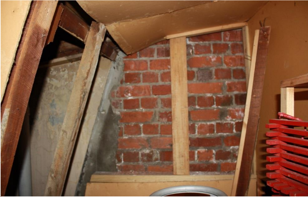
Unreinforced masonry party wall shared with the 'Pascoe's' building
