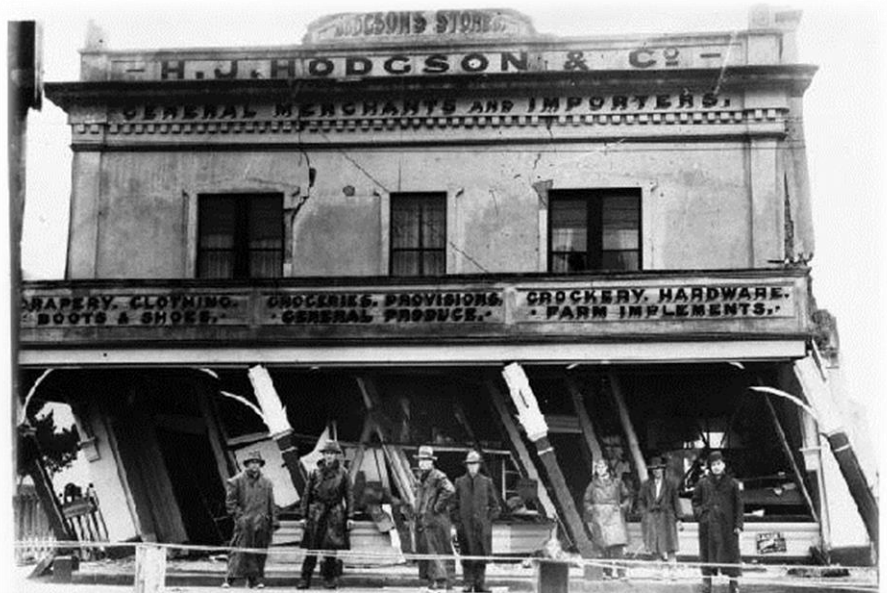
Earthquake damaged store in Murchison – H. J. Hodgson & Co.
