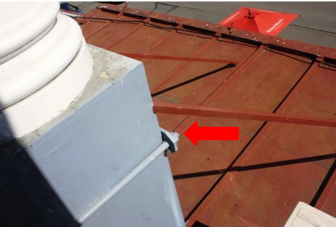
Above: Metal ties holding back the façade and tying it to an internal concrete wall
