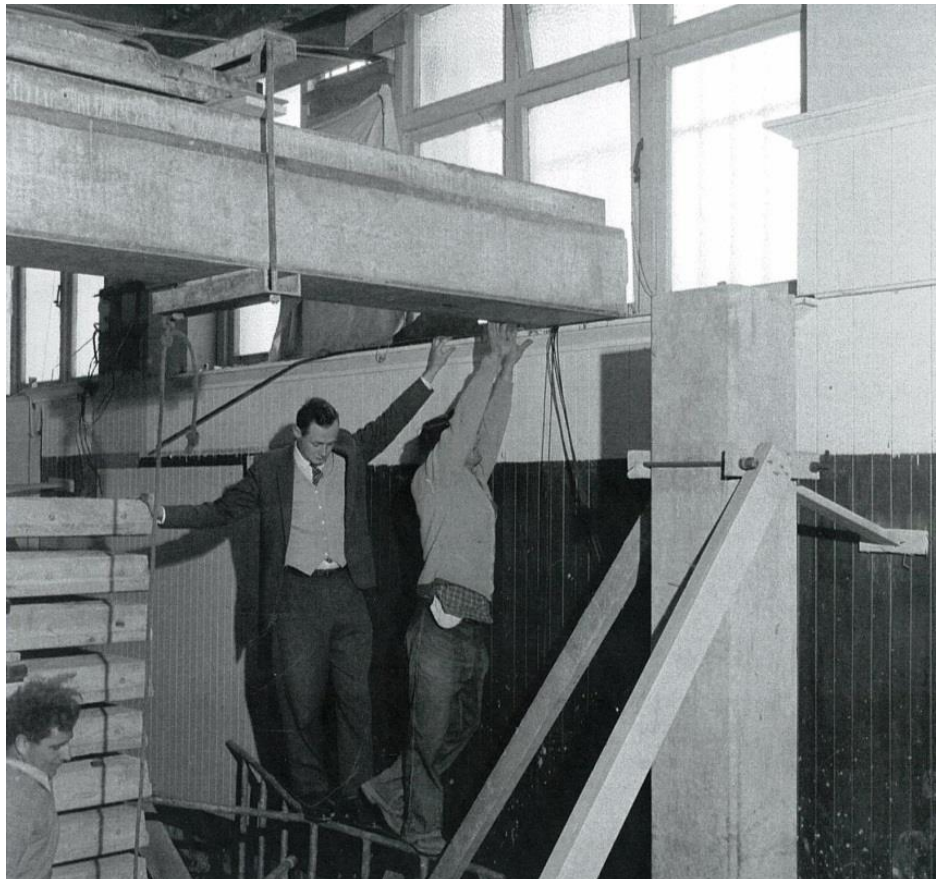
Ben Trathen helping the builder install the concrete beams
