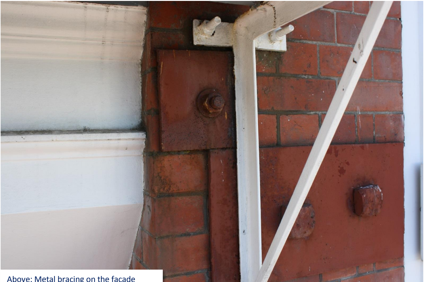
Below: Bolts & plates on the outside of the concrete wall connecting the metal ties and the front of the building
