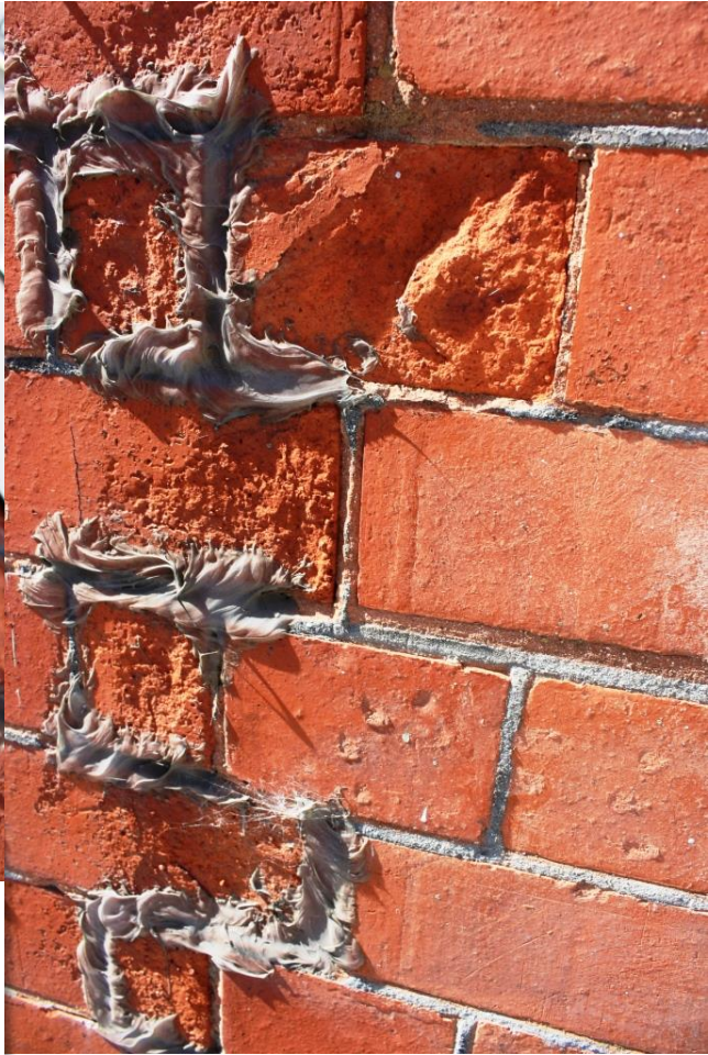
Inangahua earthquake 1968: Damage to the brick columns on the façade, very amateur repairs have been carried out with silicon to stop water penetrating and causing more damage.
